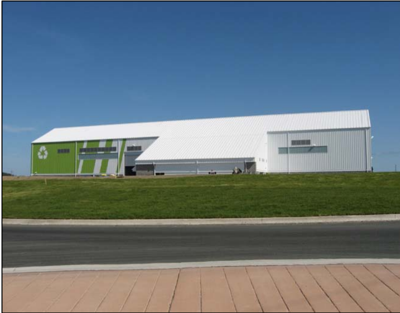
RHB Materials Recovery Facility
