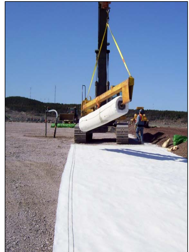
RHB Liner Installation
