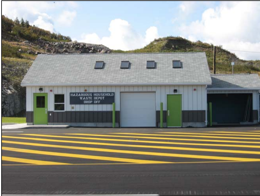
HHW Facility at Residential Drop-Off Facility
